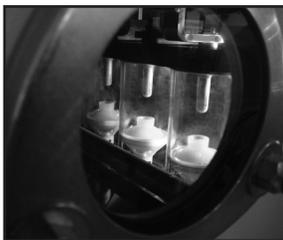
◀ Load break switch visible break.
