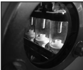
◀ Load break switch visible break.
