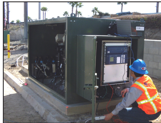
The SEL 1102 central processing unit is mounted within one of the SEL 451 relay cabinets on the side of the switch.
