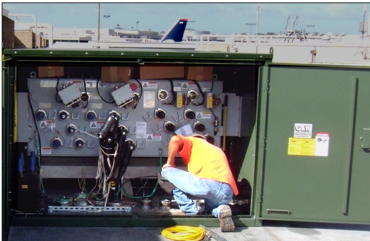
Automated multi-way switch with SEL 451 relays mounted in a side compartment.
