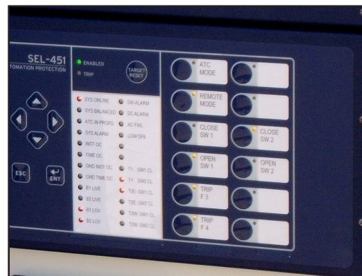
Large, clearly labeled pushbuttons provide an easy way for facilities personnel to operate individual switches safely and with confidence.
