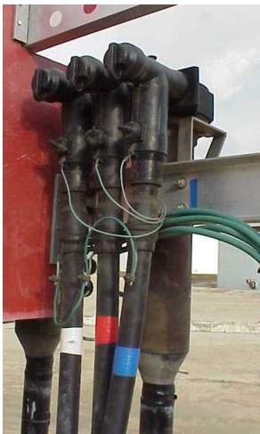
G&W's 15/25kV deadend joint in a substation application.
